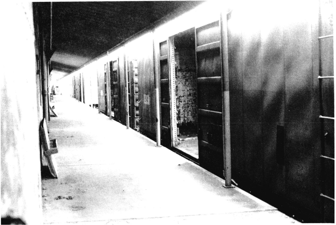
Figure 3-3.. Typical loading dock with height equal to rail car floor height.
