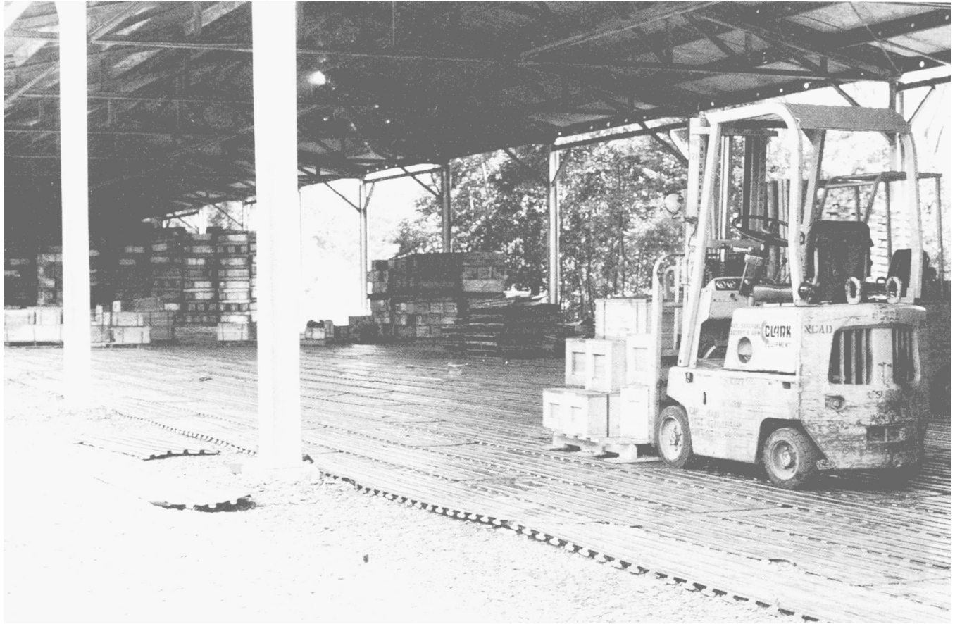
Figure 4-3. Flooring in shed area upgraded by use of steel military landing mats.
