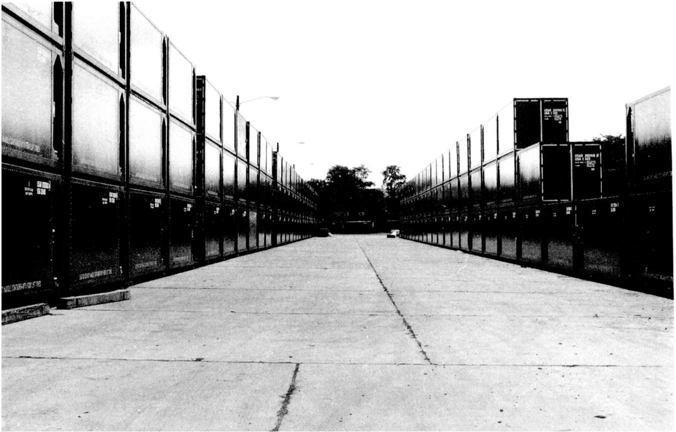
Figure 4-6. Containers stacked 3 high on concrete pavement.
